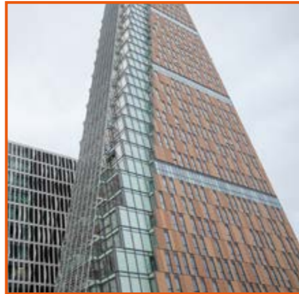
88 WOOD LANE - ONE OF THE IPO BUILDS
