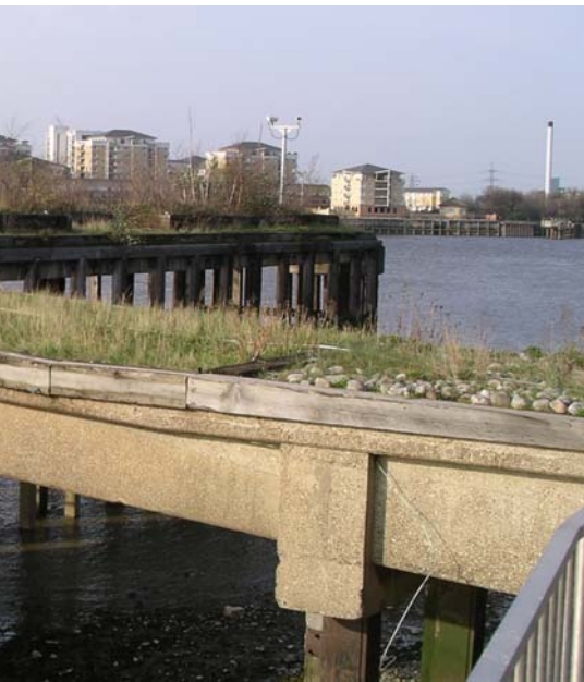
LEFT: An old jetty on the Meridian line, grassed and planted to provide wildlife habitat.
