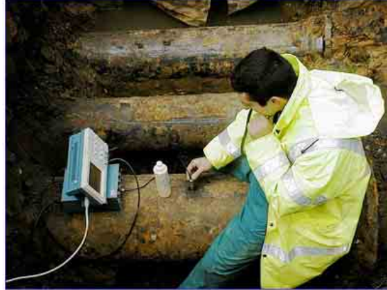
Figure 2.1: Photograph of a conventional point by point through-transmission inspection technique around a small diameter water pipe.
